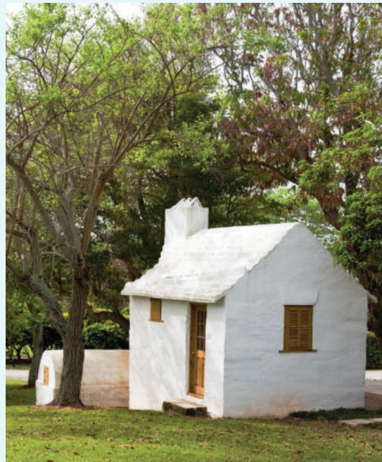
Tiny old Bermuda cottage with limestone roof - to catch water in the separate raised water tank below the house.
